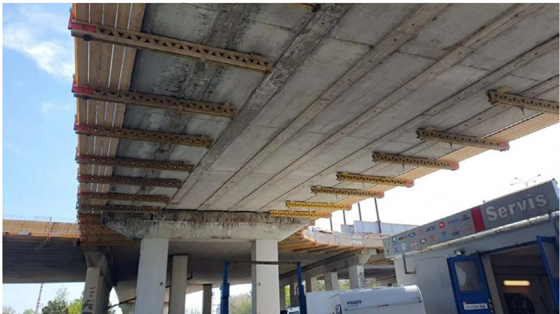
Fig. 3: Bridge span made of I-73 girders
