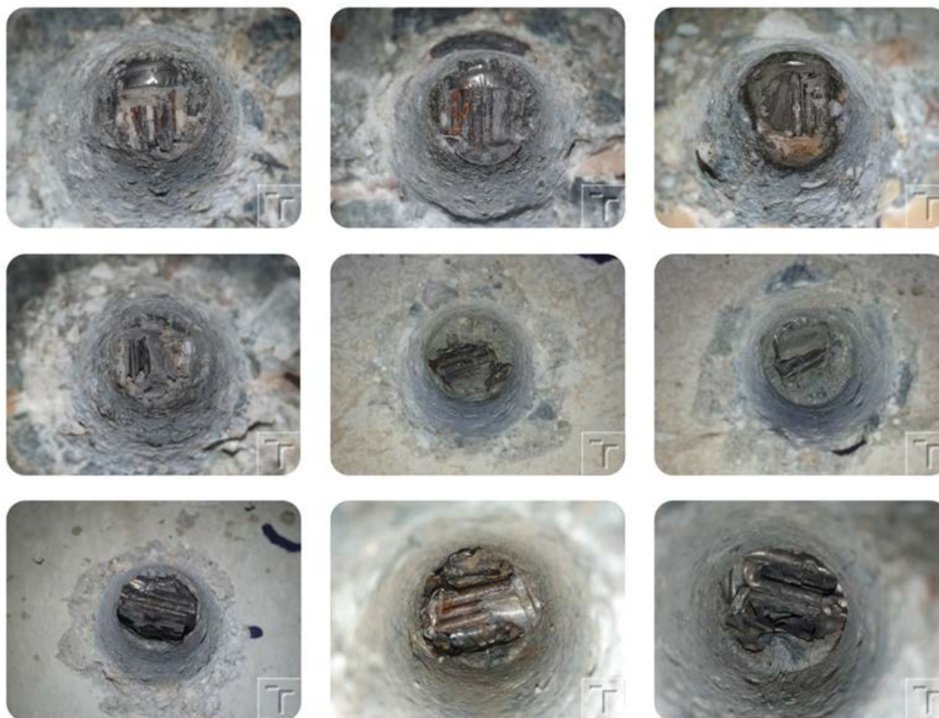
Fig. 6: Visual inspection of reinforcement in SDT probes
