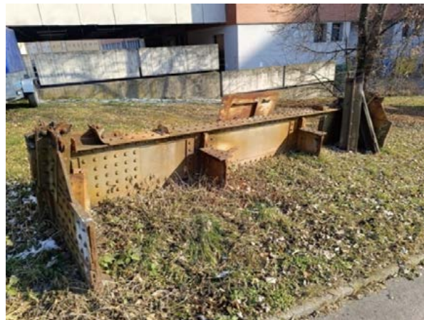
Fig. 1: Lower flange of dismantled truss structure [18].
